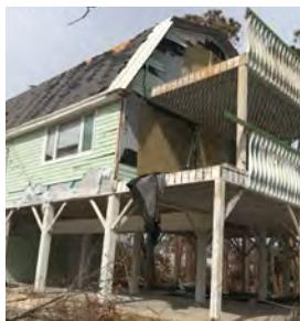
Elevated homes, common in coastal communities, will be better designed for hurricane winds using new wind load specifications in the building code. These wind load specifications were derived from hurricane field damage data and wind tunnel experimental data available in **DesignSafe**.
